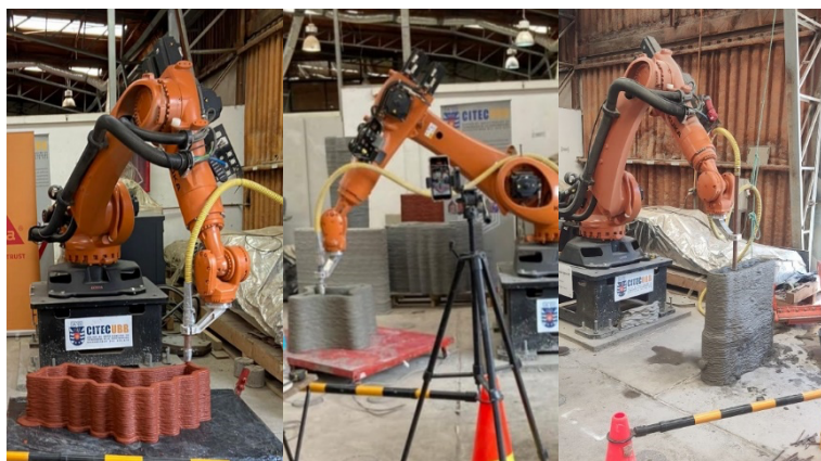
Figure 1. Example of 3D concrete elements printed with the robot used in this research.
